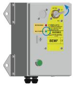
Turn the key to OFF position to switch the power off. A movement detector gives a signal to the BEMF unit once zero movement has been detected. This will illuminate a green LED. The key may now be released by pushing the green button. This key is then taken to unlock the access lock on the motor unit.
